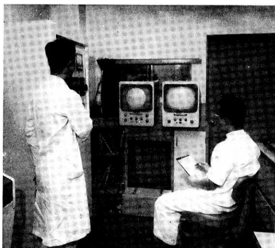
FIG. 3. The control room of the x-ray television system. There are two television monitors; the left one is for telefluoroscopy, telerontgenography and telecinorontgenography and the right one for a general view of the examination room.
